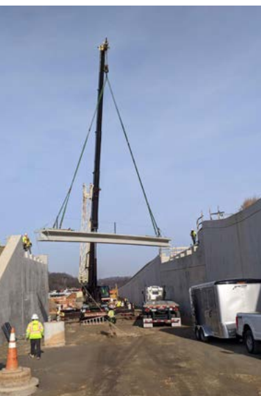
From left to right: Crews recently installed seven concrete girders for a future bridge over the light rail tracks to provide access to the Glenridge Shopping Mall in Landover Hills. Crews work on the platform and station at the Paul S. Sarbanes Transit Center in Silver Spring
