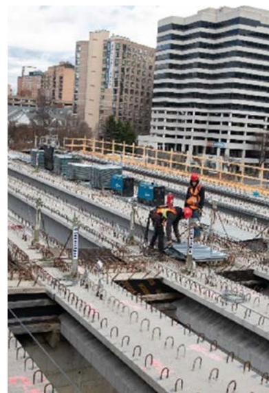
From left to right: Crews recently installed seven concrete girders for a future bridge over the light rail tracks to provide access to the Glenridge Shopping Mall in Landover Hills. Crews work on the platform and station at the Paul S. Sarbanes Transit Center in Silver Spring
