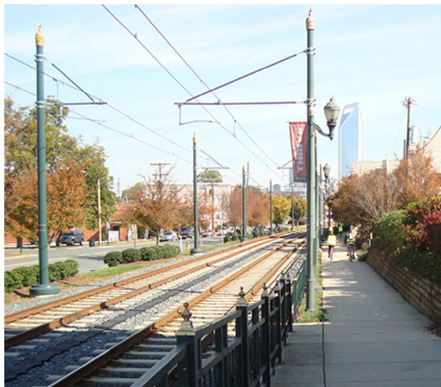
Figure 2-18. Auto Tensioned Catenary System
