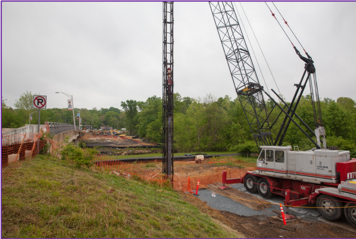
Pile driving along River Road for the foundations of the future bridge
