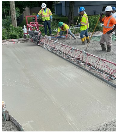
From left to right: Crews put the finishing touches on concrete holding the direct fixation track in the Plymouth Tunnel. Measuring 1,100 feet, it is the only tunnel on the Purple Line and will be home to the Manchester Place station at the tunnel's western portal. (Right) Crews place concrete for the approach slab connecting the Talbot Avenue Bridge to Grace Church Road in Woodside. Crews install a massive sand filter as part of stormwater management improvements at the University of Maryland College Park campus. The underground structure is comprised of precast concrete chambers that reduce storm surge and filter runoff through sand, removing pollutants that can negatively impact local streams.
