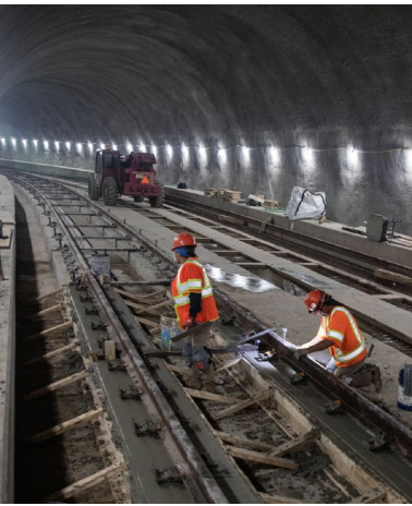
From left to right: Crews put the finishing touches on concrete holding the direct fixation track in the Plymouth Tunnel. Measuring 1,100 feet, it is the only tunnel on the Purple Line and will be home to the Manchester Place station at the tunnel's western portal. (Right) Crews place concrete for the approach slab connecting the Talbot Avenue Bridge to Grace Church Road in Woodside. Crews install a massive sand filter as part of stormwater management improvements at the University of Maryland College Park campus. The underground structure is comprised of precast concrete chambers that reduce storm surge and filter runoff through sand, removing pollutants that can negatively impact local streams.
